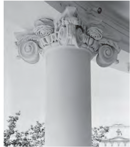
Capital of a Column on the Truman Balcony
