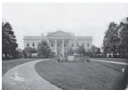
Historic Photo Showing North Portico
