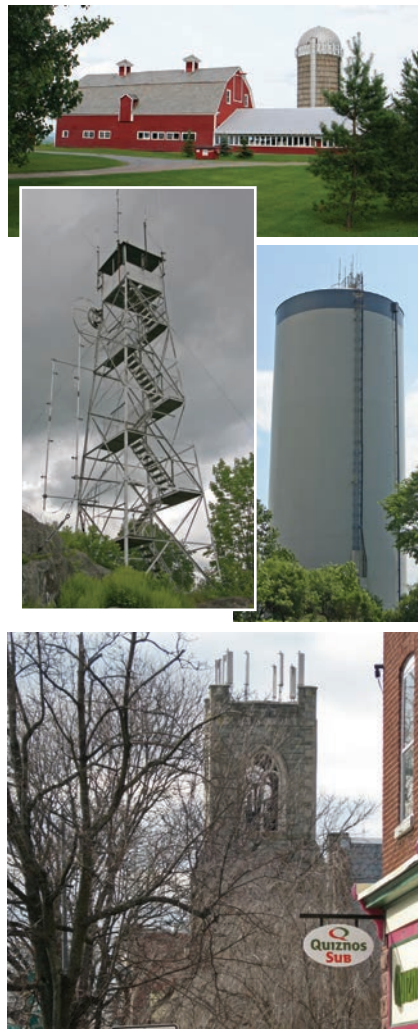
Communications antennae have been placed on a silo in Burlington, Vermont, a fire tower in Moriah, New York, a water tower in South Burlington, Vermont, and a church steeple in Bloomsburg, Pennsylvania.
